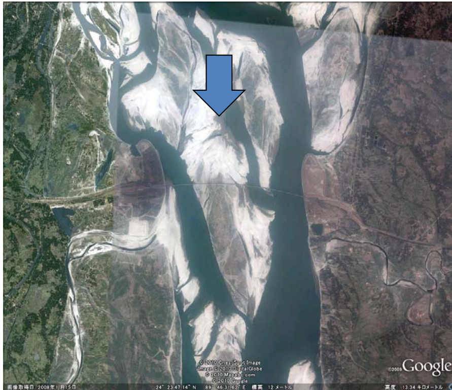
Jamuna Bridge in Bangladesh
