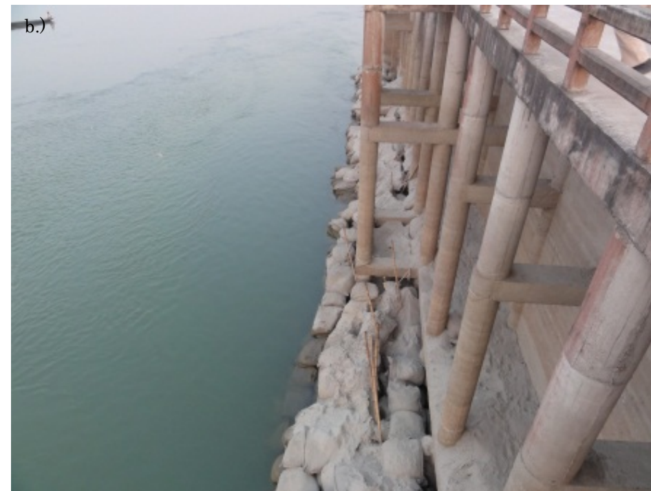
Photo 4a) Enayetpur Spur on Jamuna River, 4b) geobag reinforcement around pilings of semi-permeable spur dike.
